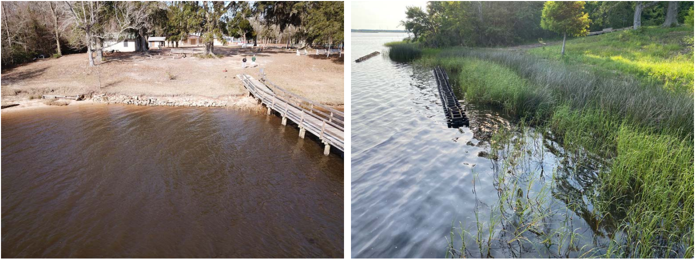
FIGURE 1. A Biloxi, Mississippi, site is shown before (2018) and after (2021) installation of a living shoreline. Photo Credit: Eric Sparks
