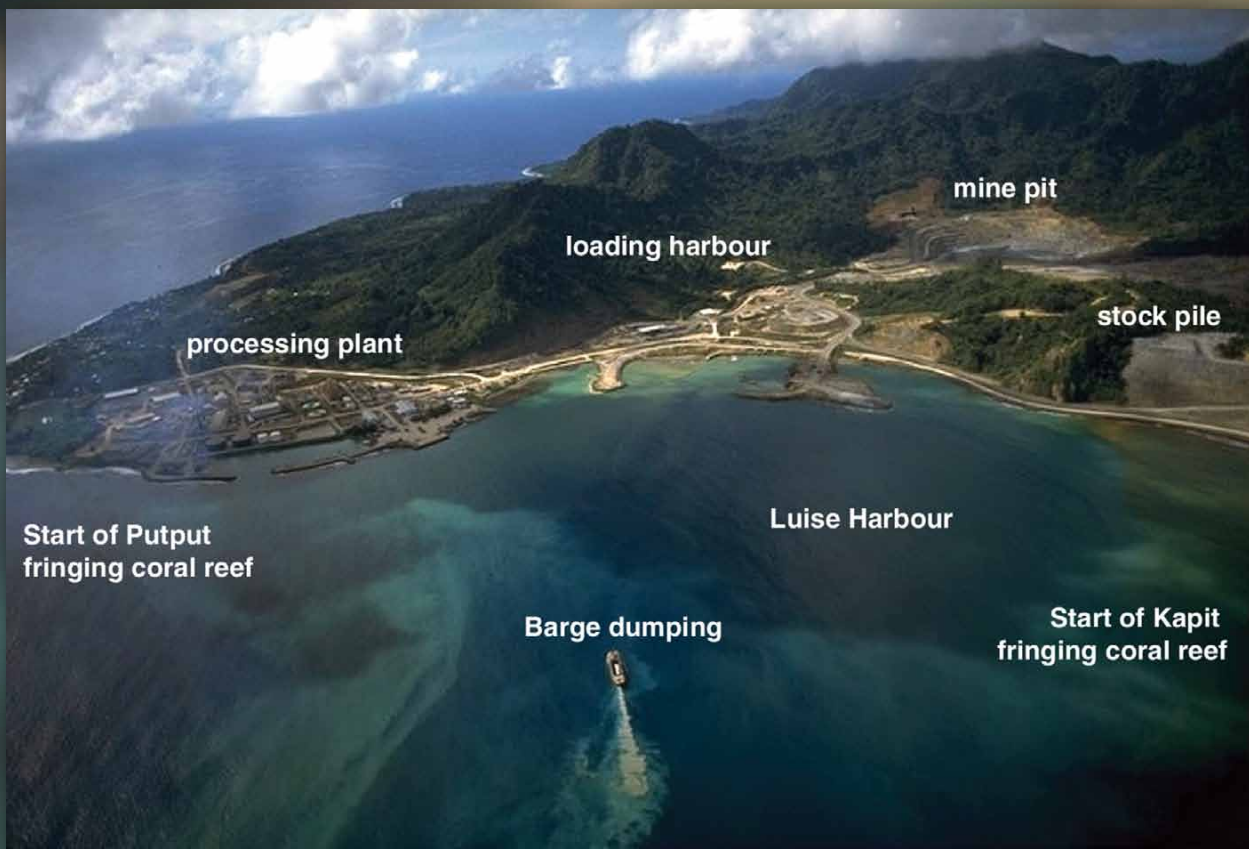
Luise Harbor with dumping barge in the foreground. Photo courtesy of Lihir Management Company
