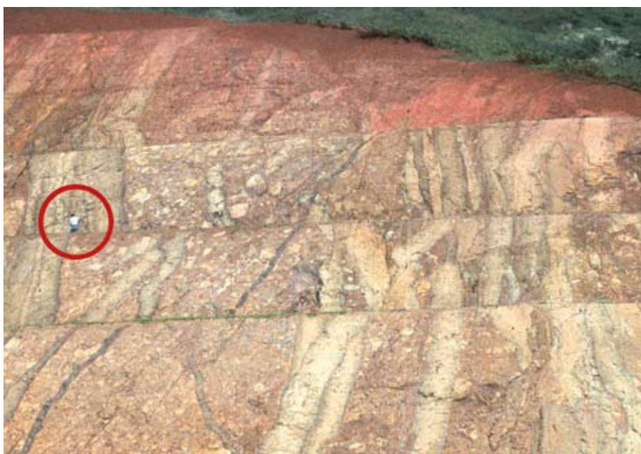
Figure 1. Dike intrusions (vertical and slanted features) into the Koolau volcanic shield, Oahu, Hawai`i. Photo taken during road construction where the road cut is defined by three, near-horizontal "staircase" steps. A person on the second terrace (circled) offers a scale.
